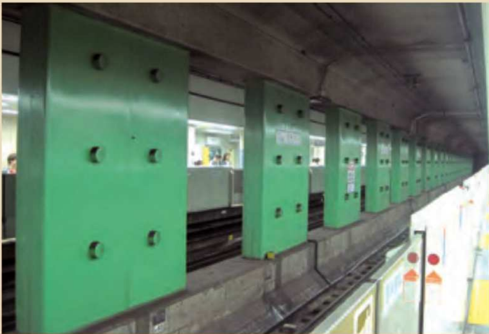
Platform Column Reinforcement
