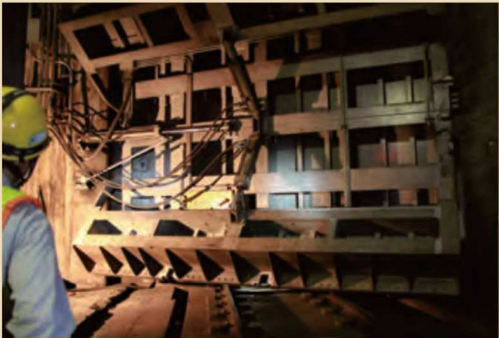
Waterproof Gates (In Tunnels)
