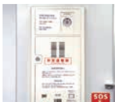
▲Emergency communicator and emergency stop button
