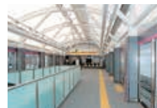
▲Platform doors and tactile paving
