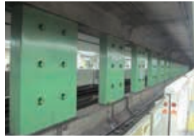
▲ Reinforced station pillars
