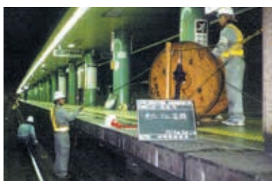
▲ Installing optical fiber cables
